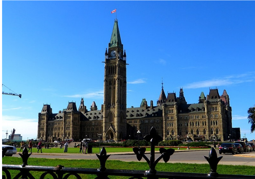
Centre Block, Canadian Parliament Buildings – Built with Tyndall Limestone Credit: Ken Lund , Creative Commons Attribution-Share Alike 2.0 Generic license
